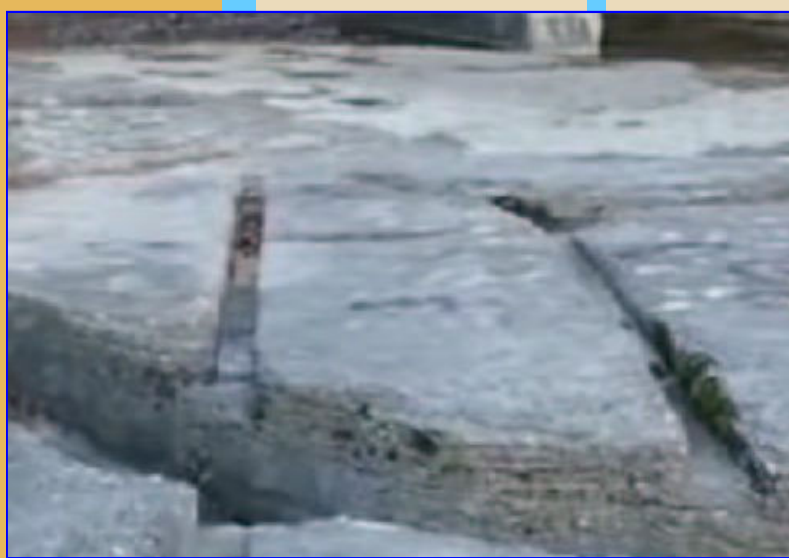
Fig. 4. A fortuitous cross-section of the tracks. It is located right at the edge of the 1' break: 5' apart, rim-to-rim (confirmed by Google Earth), 2.5"-5.5" in depth and flat bottomed, straight down sides. In other words, they appear in every way to be cut into the rock surface artificially.
