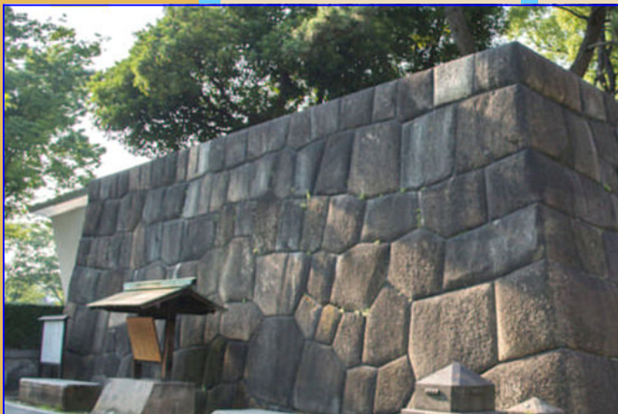
Fig. 3. Similar, though not as precise as the stonework at Cuzco, is that of Edo Castle in Tokyo, Japan. It shows what may yet be the mysterious phenomenon of stone softening technique. Wikimedia Commons.
