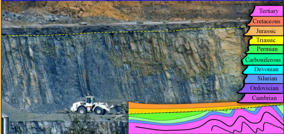
Fig. 3. Typical ancient unconformity at Roche Blain quarry. Very flat surface depleted of differential erosion. Paleozoic layers were folded during the Hercynian orogeny; truncated during the Triassic; buried under Jurassic sediments.
