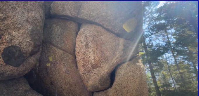
Fig. 4. Polygonal shaped-to-fit Wall section, opposite Sage Wall on a ruined section. It's what's holding up the path in front of Sage Wall, as a retaining wall. Photo by Will Brown.
