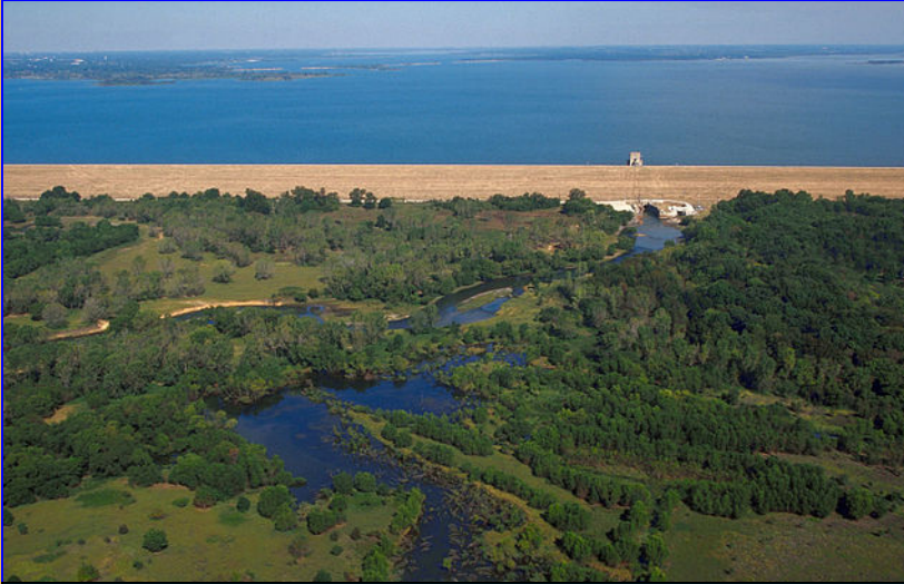
Fig. 2. Aerial view of Lewisville Lake and Dam on the Elm Fork of the Trinity River in Denton County, Texas, USA. The lake is located near the town of Lewisville about 20 miles (32 km) north of Dallas. Photo: U.S. Army Corps of Engineers, crop, Wikimedia Commons.
